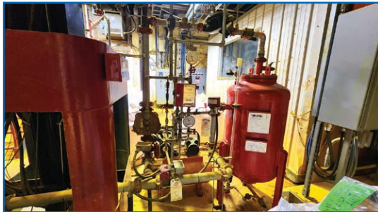
2019 VIKING VFT PRESSURE PROPORTIONING SYSTEM
